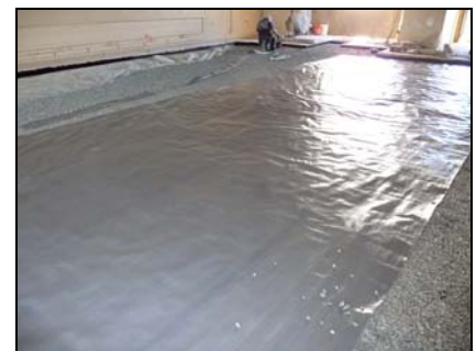
Laying out Geo-Seal BASE Layer
