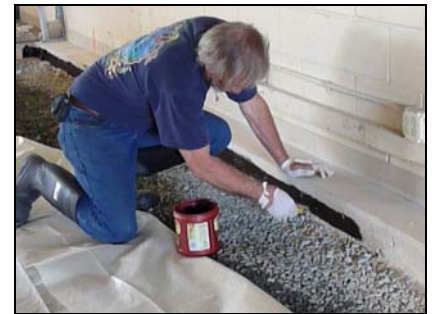
Vertical Termination Preparation
