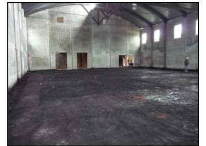
Geo-Seal spray-applied, CORE layer
