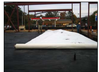
Geo-Seal BOND layer application
