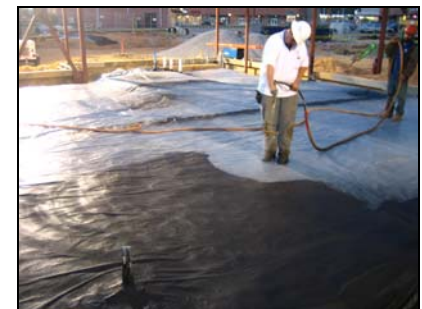
Geo-Seal spray-applied CORE layer application
