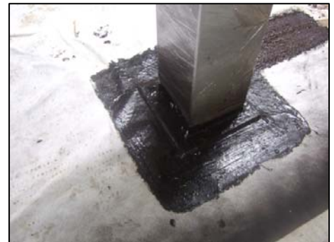
Sealing around Steel Stanchion
