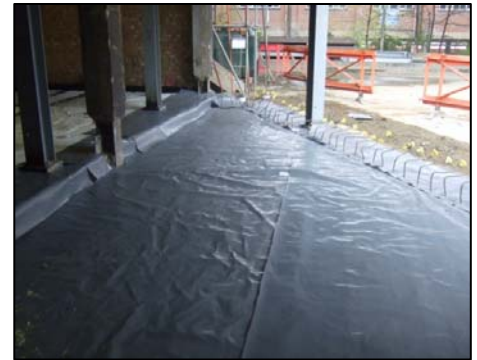
Placing the BOND Layer
