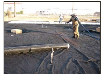
Geo-Seal Core Installation
