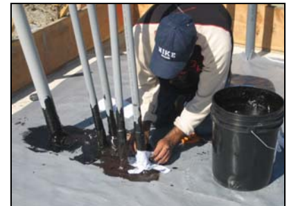
Sealing Penetration Cluster
