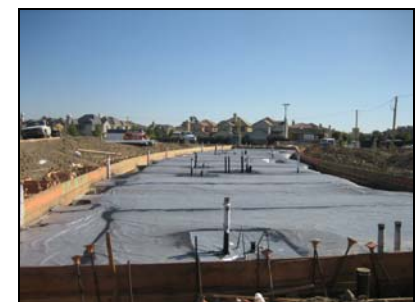
Completed Geo-Seal Installation
