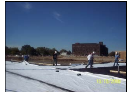
Installing the Geo-Seal BOND Layer
