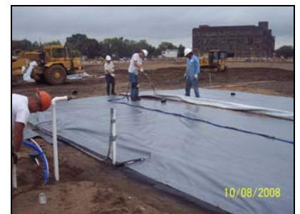
Seaming the Geo-Seal BASE
